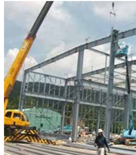
工場新築工事
